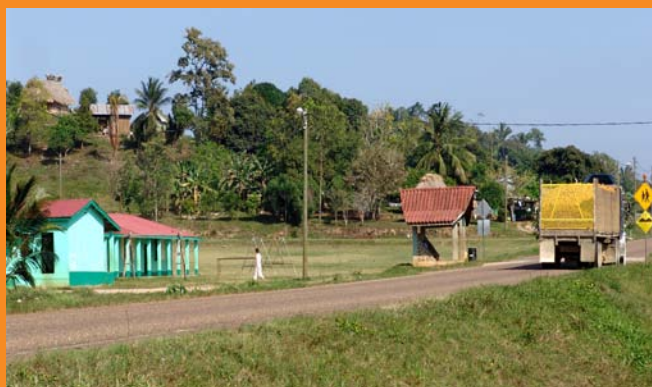
The second phase of the project to electrify Armenia Village, along the Hummingbird Highway, was completed in 2004, under the Power III Rural Electrification Project.
