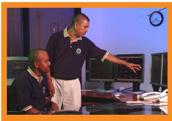
Employees in the Dispatch Center monitoring the Transmission and Distribution System.
