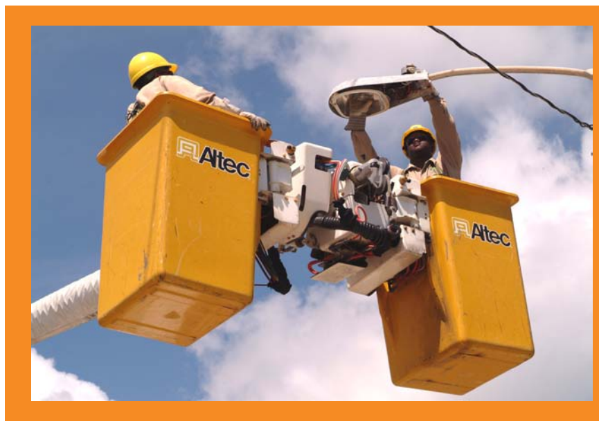
BEL Linemen replacing a street light as part of an aggressive effort to identify and correct faulty street lights.
